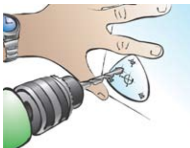
Drill hole for sensor wire.
