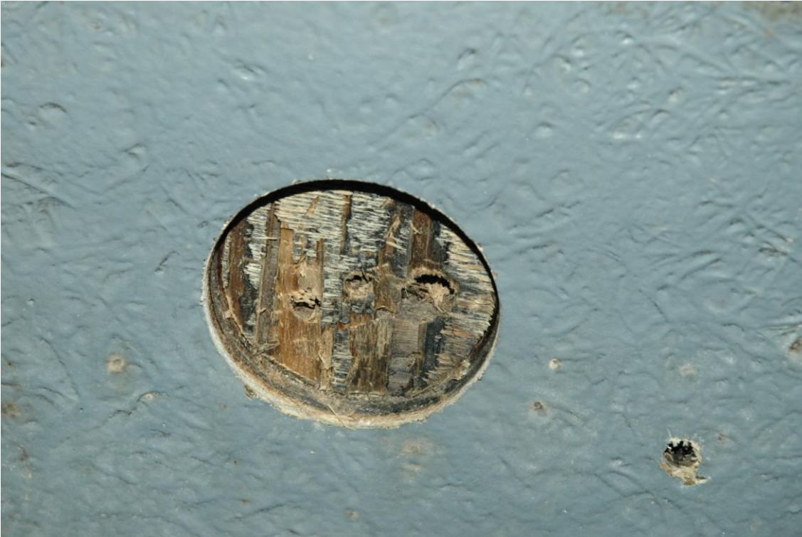
Figure 24 Rotted stringer from leaking shower or side windows.
