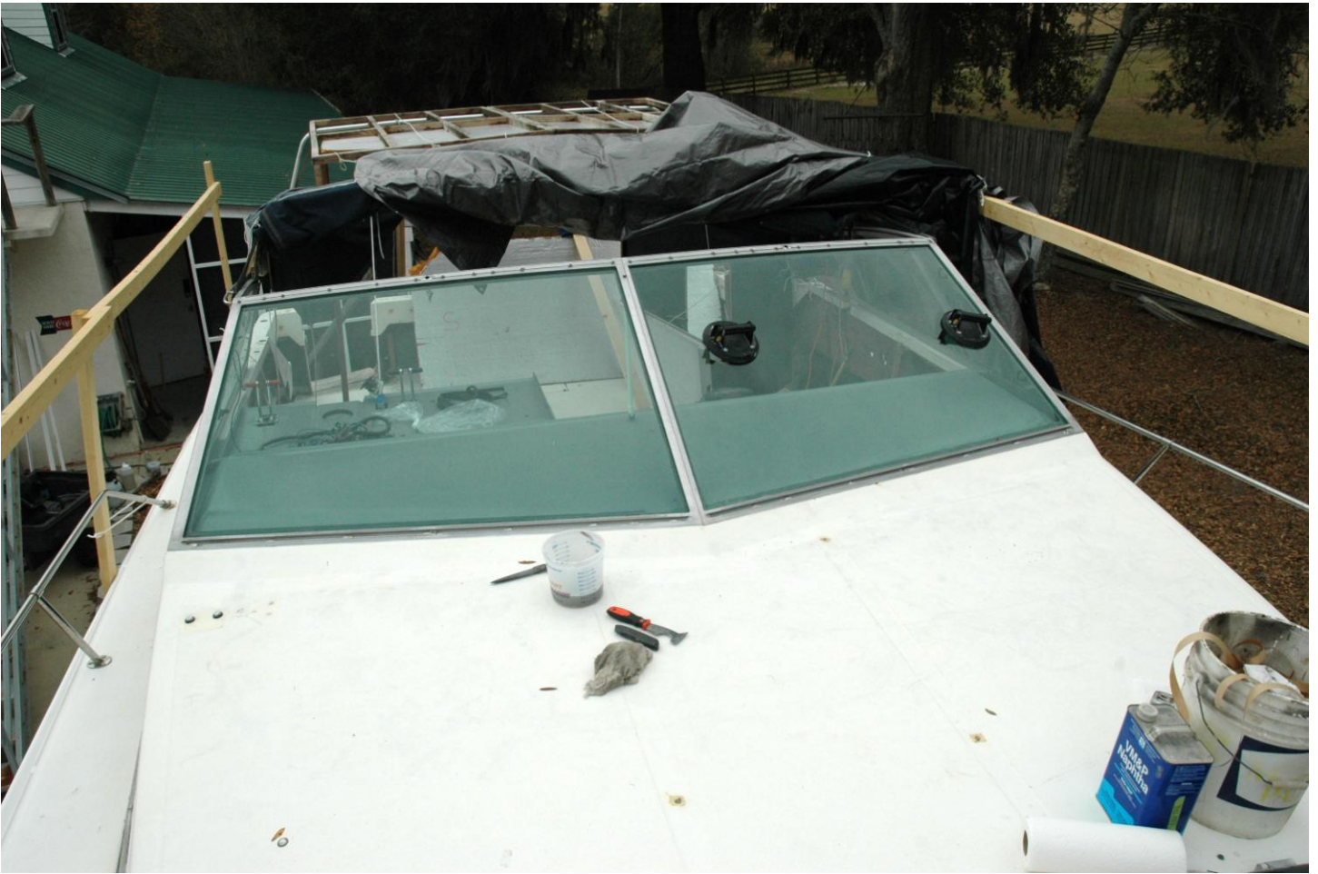
Figure 15 Glass is really big. NEVER lay flat! Always on edge!
