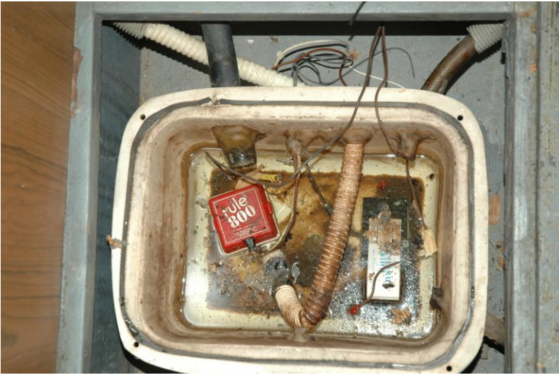
Figure 8 Shower Sump after rebuild
